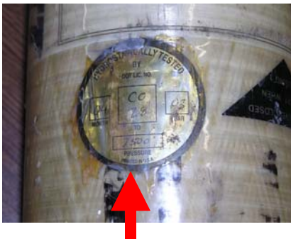
Hydrostatic Testing Label
